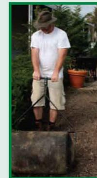
**8. Roll the area** with a lawn roller one-third full of water to firm and settle the surface. Low spots should be filled to match the surrounding grade surface. If time permits, allow area to settle further with rainfall or by applying irrigation.
